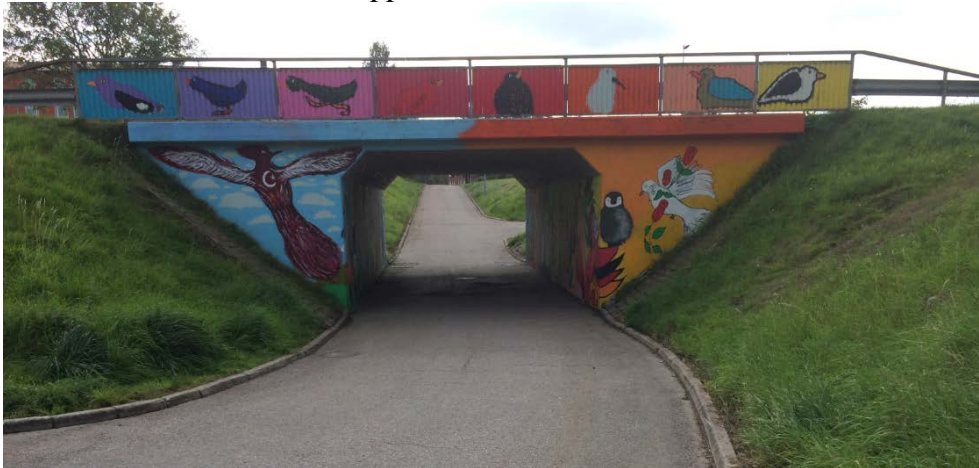
GC-tunnel under Groppbrovägen
